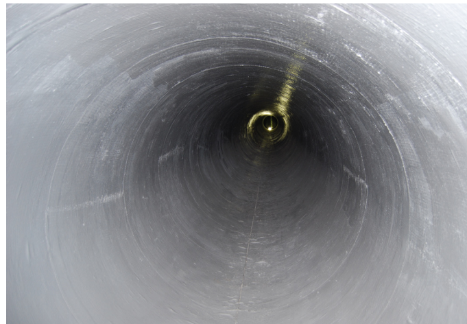
Fig. 6: Completed lining, including gray top coat, prior to testing
