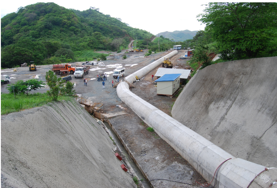
Fig. 1: Above ground segment of the El Encanto penstock
